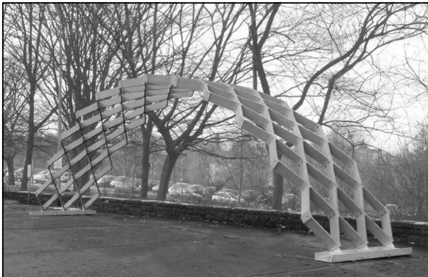
Prototype of a diamond-shaped lattice grid. Textile Reinforced Concrete (TRC) is a composite material made of open-meshed textile structures and a fine-grained concrete. Comparable to steel reinforcement the textile fabric bears the tensile forces released by the cracking of the concrete. Only a minimal concrete cover is required for the bond of the textile fabrics. Thus, the application of TRC leads to the design of filigree and lightweight concrete structures with high durability and high quality surfaces. In recent years, TRC has been successfully employed for the production of ventilated façade systems. Current investigations enlarge the application range of TRC to façade systems with large spans and load-bearing structures. In this paper, the investigations on self-supporting and structural sandwich panels regarding production methods, results of bending and shear tests, tests on sound insulation and fire resistance as well as first prototypes of slender frames and shell elements are presented [8].
